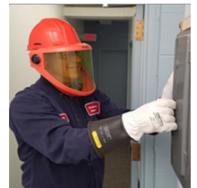
Roger Sroka, Electrician, inspecting a fuse box.
