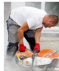
Work Conducted Without Water Control
