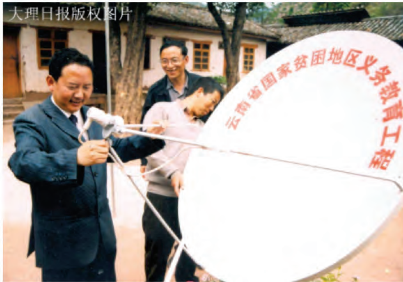
Figure A2: Installation of Satellite Receiving Systems
