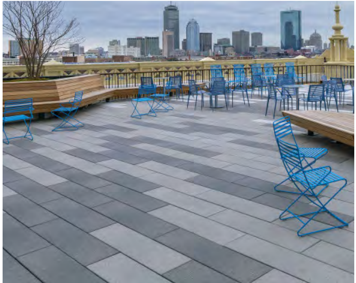
Pavers on roof deck example in Boston
