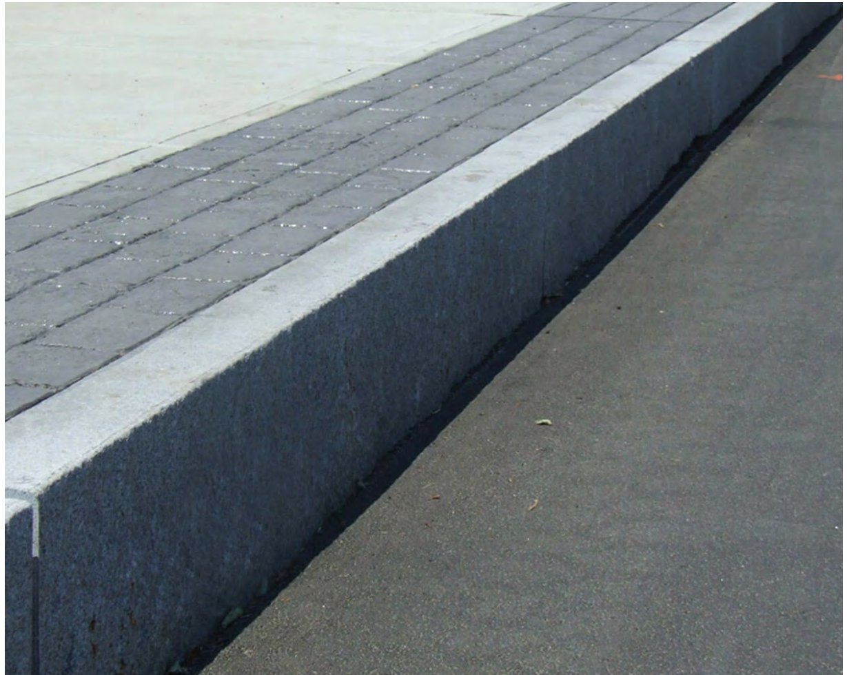
Raised Granite Curb at Campus Street
