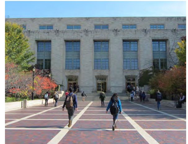
Ironspot bricks at the Tech entry plaza
