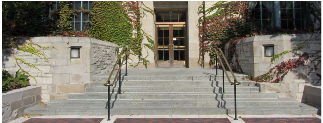
Granite stair at Tech entrance
