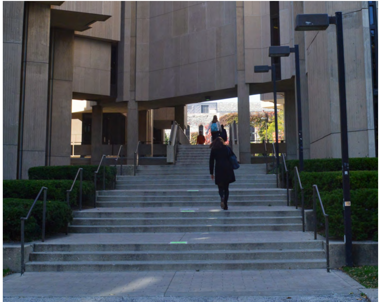
Concrete stair at the University Main Library
