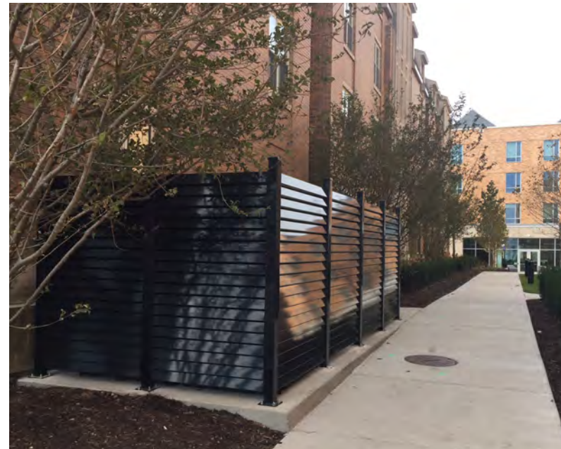
Metal refuse site enclosure at 560 Lincoln Student Residence
