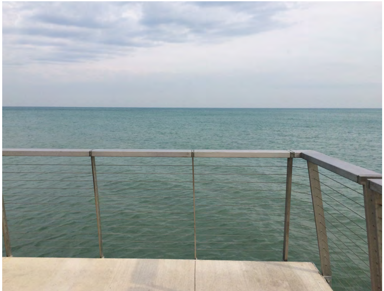
Cable guardrail along the Lakefront at the Bienen School of Music landscape
