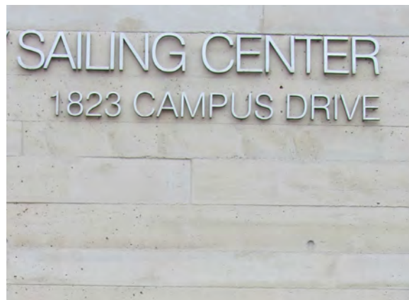
The Northwestern Sailing Center has a board form finish that is compatible with the look and feel of the Indiana limestone used in campus buildings
