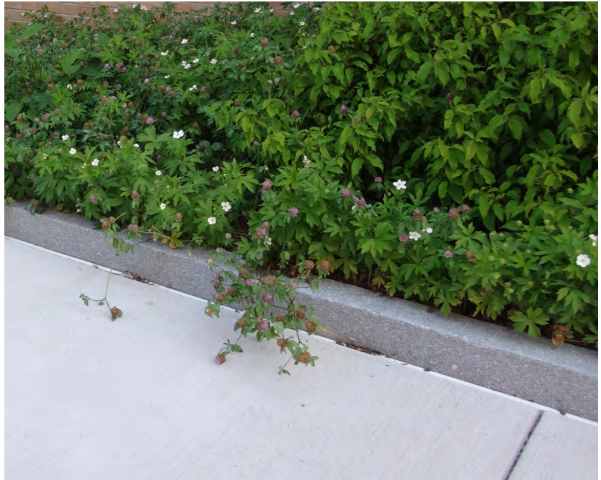
Low raised granite curb at planting bed
