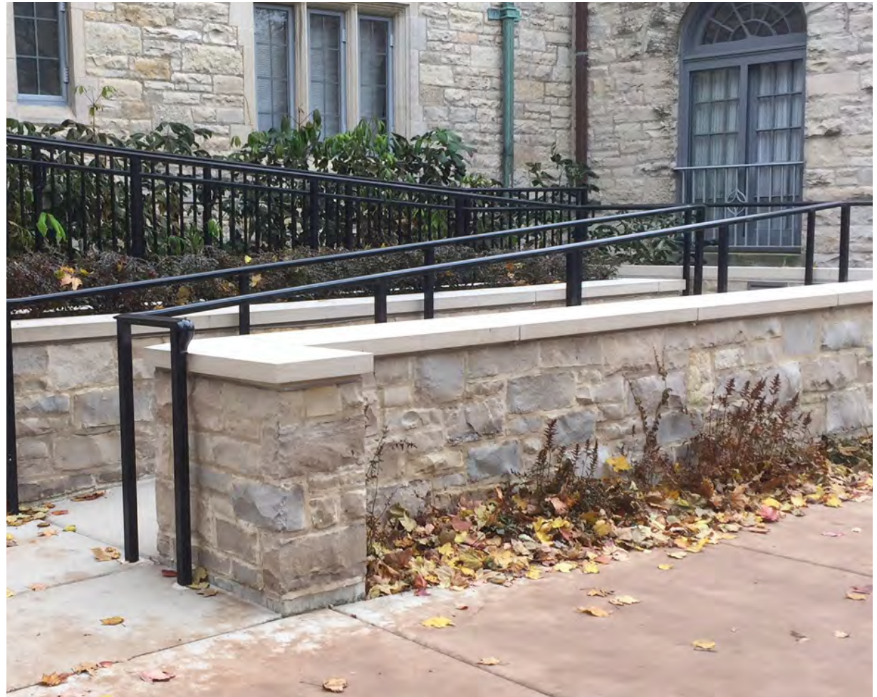
Existing limestone wall at Acessibility ramp - Sorority Quads at South Campus
