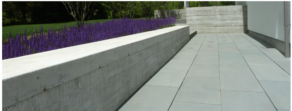
Concrete seat wall with a board form finish
