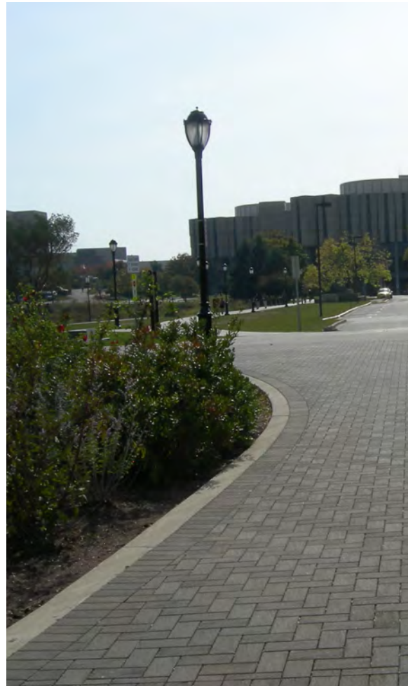
Flush curb edging at unit pavers
