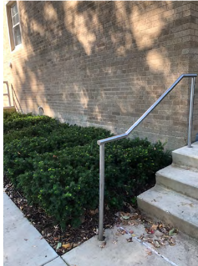
Stainless Steel Handrail at Shephard Hall
