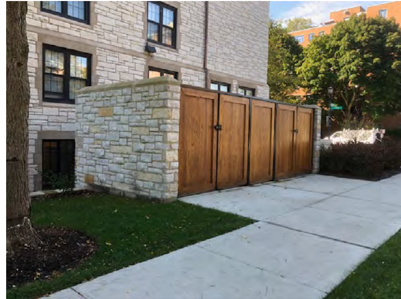
Architectural site wall screen's service area at Willard Residential College. Where possible, integrate screen wall with adjacent architecture
