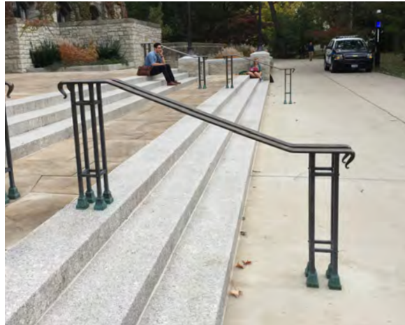
Handrails at Deering Library stairs are ornamental and compatible with the character and materials of the historic architecture.
